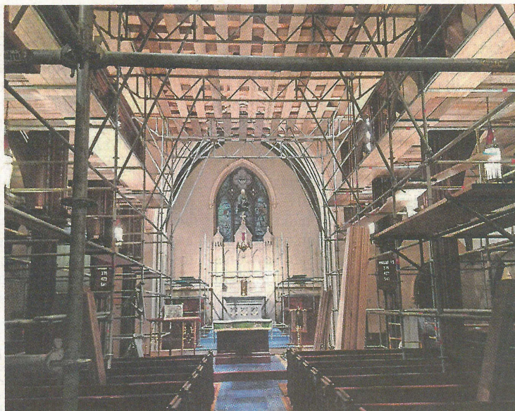
The church nave and altar underwent renovation in 2015.
